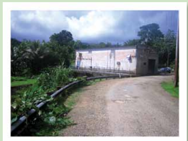
Photograph 4 - Nanipil hydro, 1.7 megawatts, generation is very compromised by a limited water resource supplying potable water for Kolonia also.
