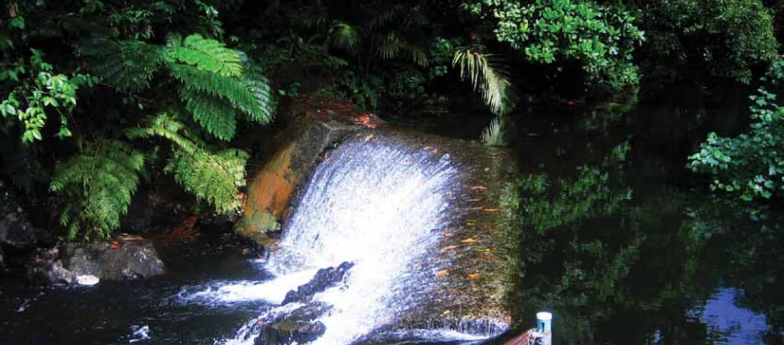
Nanpil stream water supply intake weir
