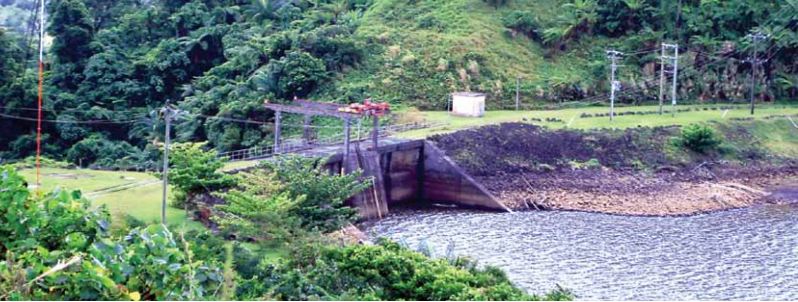
Apullio Hydro dam
