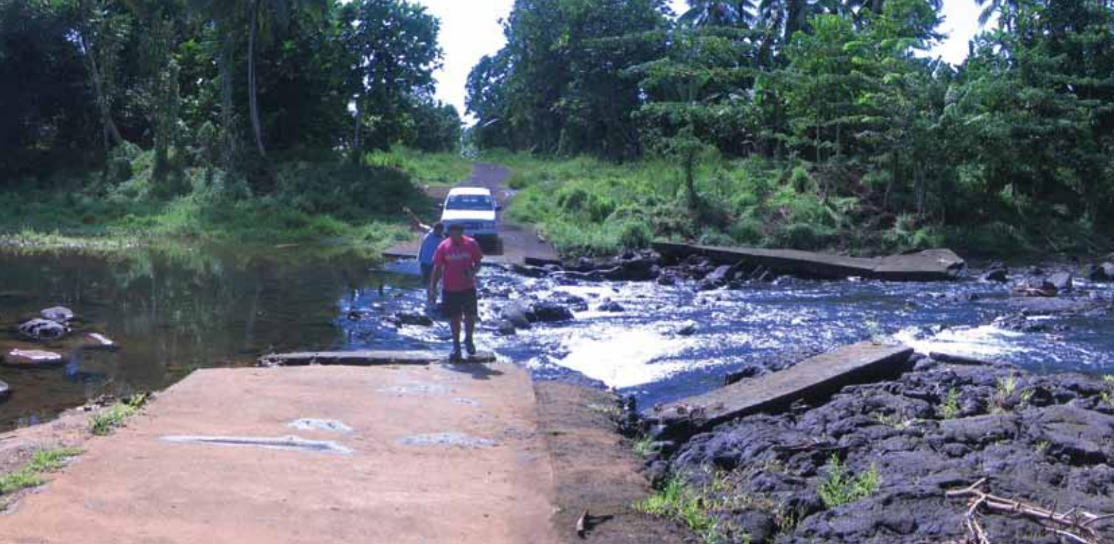
Concrete road crossing, Sili River, Savaii Island
