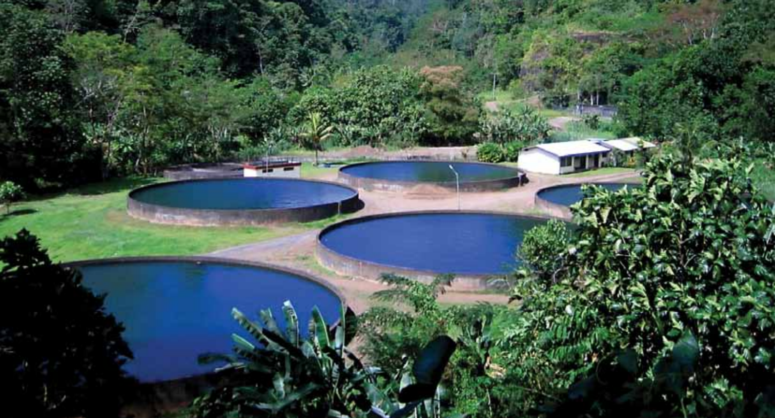
Samoa Water Authority water treatment plant at Alaoa east
