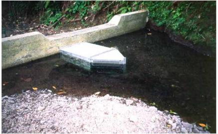
Concrete encased intake mouth to exclude leaves and debris
