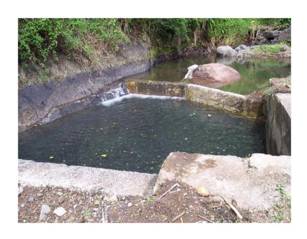
Filtration at this intake at Tupapa was simple by use of fibre sheet through which the water passes
