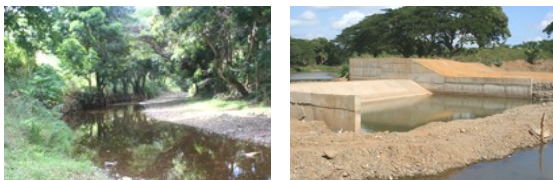
Fig. 4: Left : Typical upper catchment behind Nadi Town. Clear tributaries approaching the major sugar cane growing areas. Right : Reconstruction of gabion supports and river bank surrounding the small check dam designed to reduce high flow periods and back-up water for drip irrigation behind Nadi Town.
