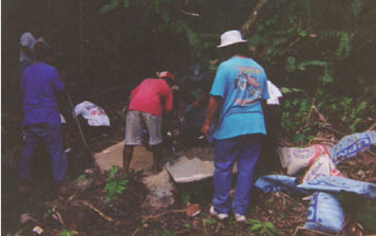
... and its construction.
