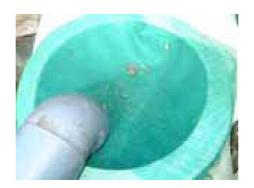
Alternatively, the downpipe from the roof could enter the tank through an **appropriately** sized hole at the top of the tank with the filtration screen at the entrance to the downpipe from the gutter.
