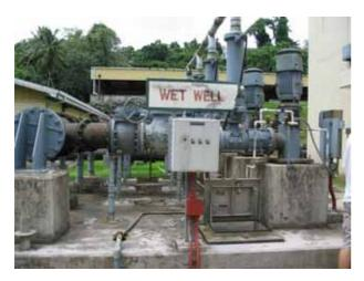
Photo: 3 Water from the two sources is collected at the Wet Well.
