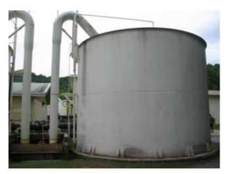
Photo: 4 Automatic Gravity Valve-less filters
