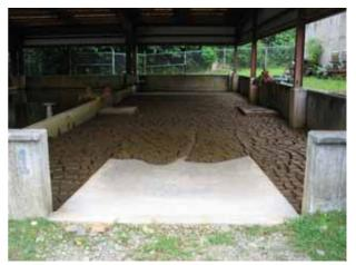
Photo: 6 Sludge drying bed
