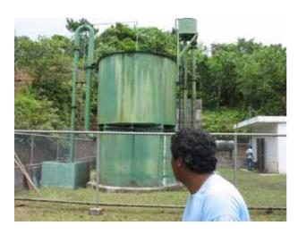
Photo: 7 Treatment plant with an AGV filter in the foreground and the typical vegetation around the catchment in the background)
