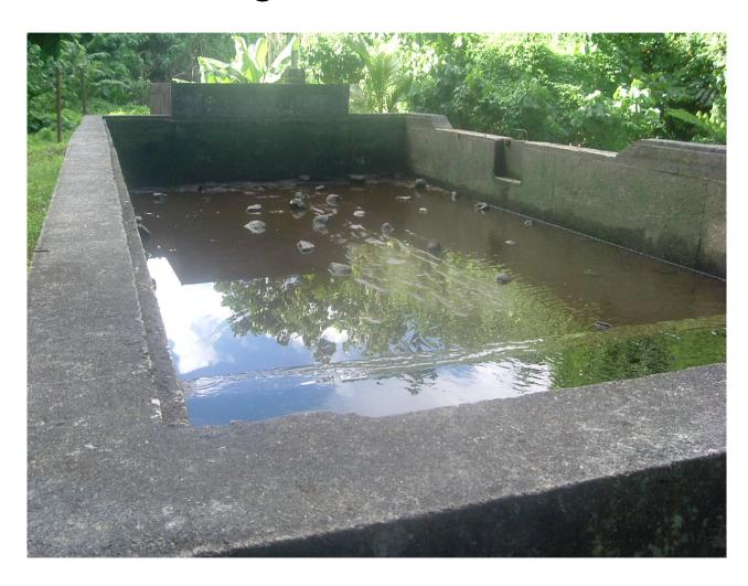
Avatiu water intake- pipes are laid under the sand for filtration purpose. The intake dries
