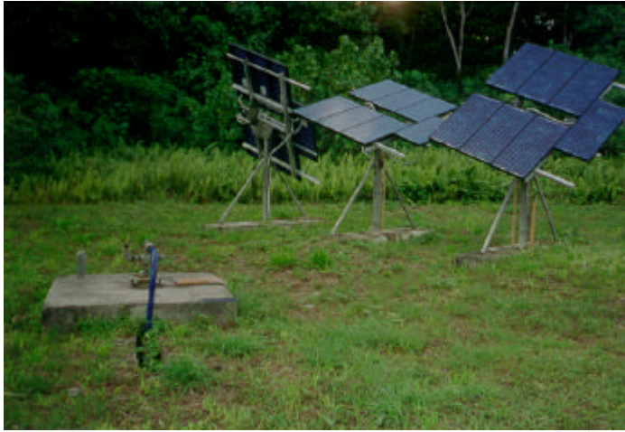
Figure 9: Makefu solar powered bore hole pump
