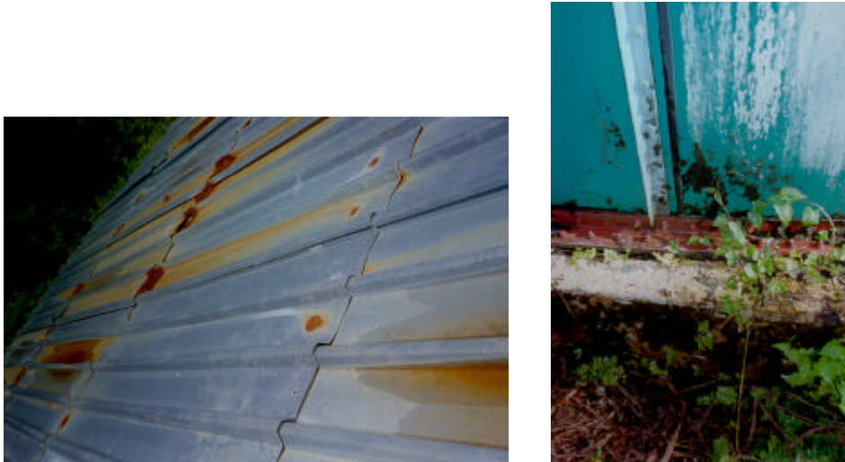
Figure 13: Rusty tank roof in Toi and leaking base on Alofi North tank
