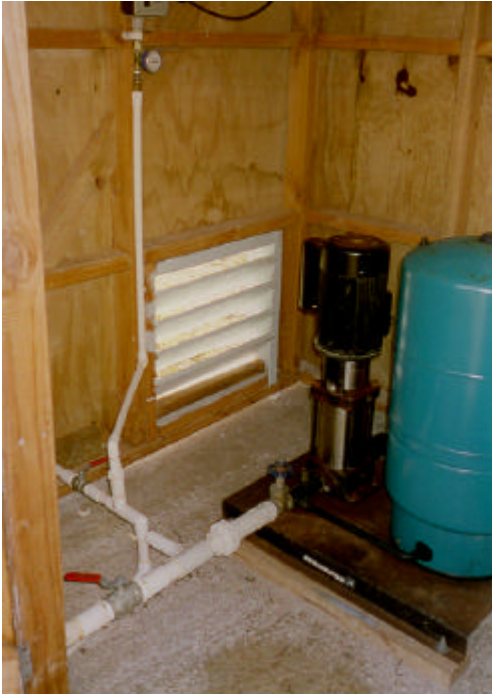
Figure 10: Pressure pump maintaining 15-30 psi pressure range in village distribution system
