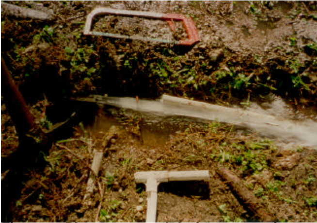
Figure 7: Pipe punctured during excavation
