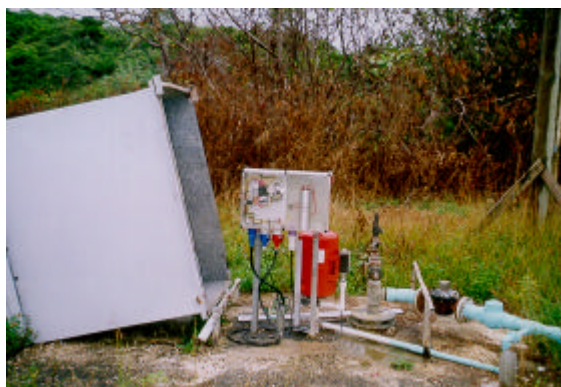
Figure 8: Liku borehole, pump, switchboard, and bulk flow meter
