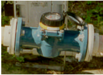
Figure 17: Bulk flow meter
