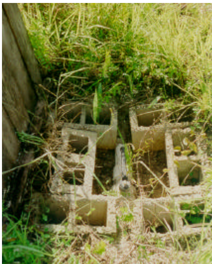
Figure 15: Valve along main in Alofi South
