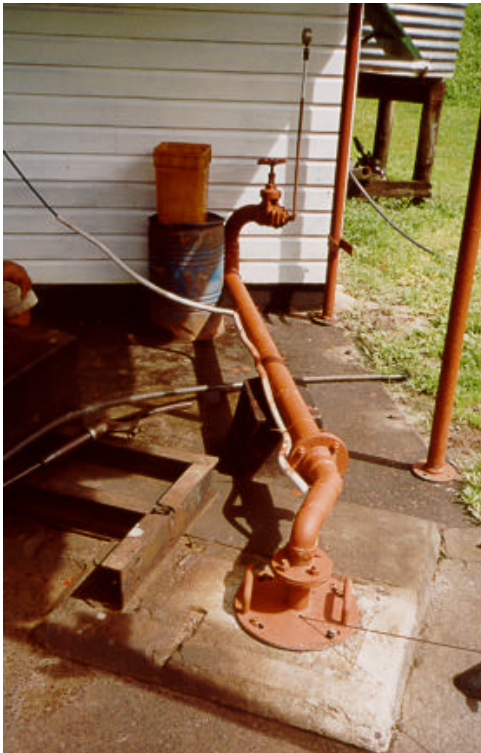
Picture 1: Motusa borehole. Bore pipe leading into the pump house is painted red to protect it from the sun.
