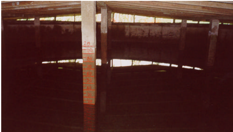
Picture 8: Inside the Motusa tank. The water level is indicated from the red markings on the support. The maximum water level is 2 m. The slight elevation of the roof is apparent.
