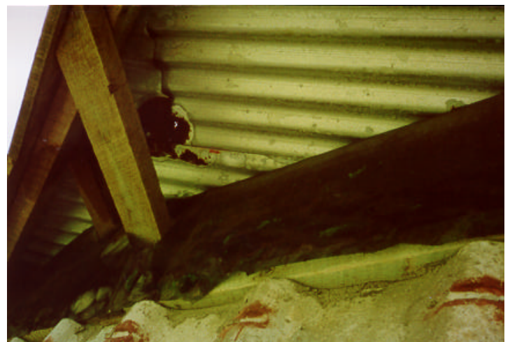
Picture 7: A rust hole through the roof of the Lepjea tank. The black mesh to keep pests out of the tank is dirty, torn and sagging between its supports.
