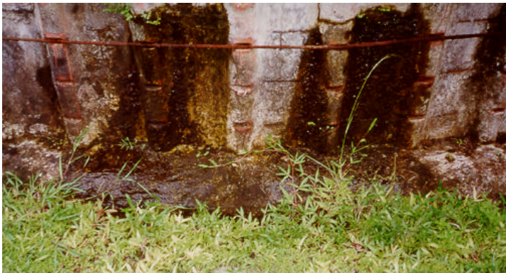
Picture 6: The leaking base of the Motusa tank. Small cracks and fissures are evident from the brown stains. The poor condition of the reinforced concrete tank is evident. Many of the reinforcements have rusted away.
