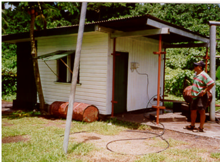
Picture 3: The Lepjea diesel powered bore pump and control panel. The pump was installed in late 1999. The control panel is manually operated by the site Warden. The pump will automatically shut down when there is over 4 ft (1.2 m) of drawdown in the groundwater level.
