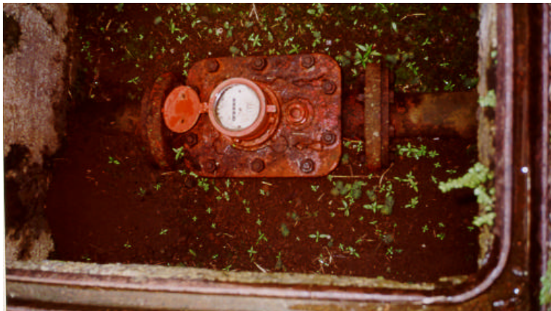
Picture 9: The bulk flow meter coming from the Ahau/Matusa tank. Readings are taken every day to give an idea of user consumption.
